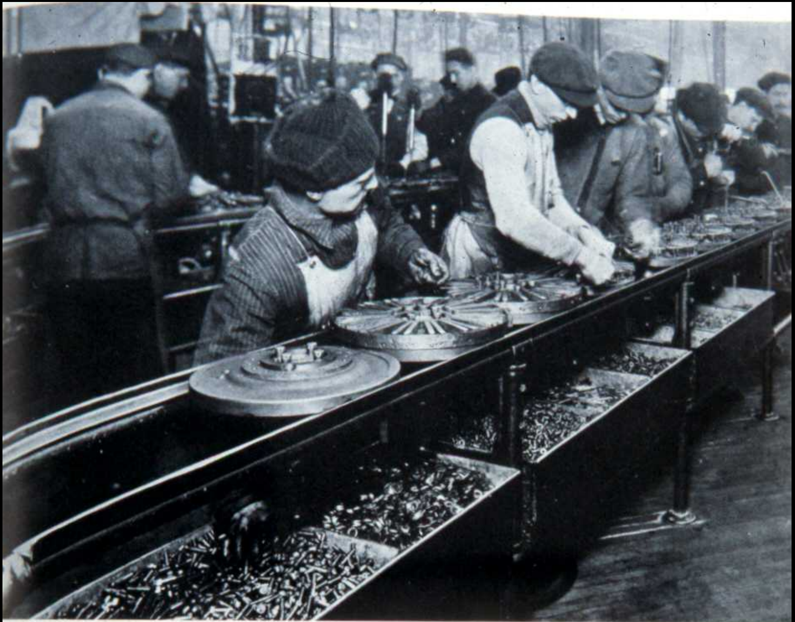
The first moving assembly. The magneto line, Highland Park, 1913
