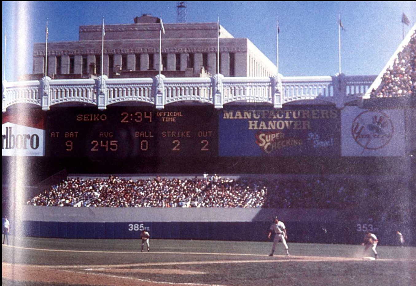
New York City's renovation of Yankee Stadium in mid-70s
